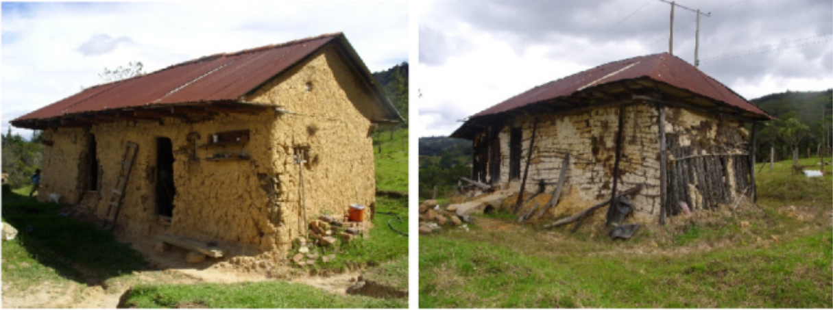
Figure 51: Wattle and Daub wall Source : MATERIALITY OF RURAL VERNACULAR HOUSING IN THE ANDEAN HIGHLANDS OF COLOMBIA: ENVIRONMENT AND BUILDING SYSTEMS www.witpress.com , ISSN 1746-4498 (on-line)
