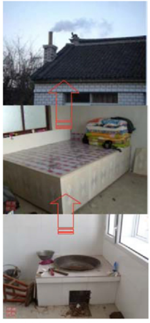
Figure 37: Kang system chimney system
