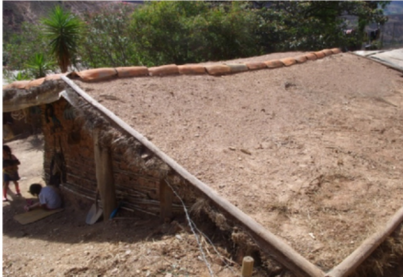
Figure 54: Straw roof Source : MATERIALITY OF RURAL VERNACULAR HOUSING IN THE ANDEAN HIGHLANDS OF COLOMBIA: ENVIRONMENT AND BUILDING SYSTEMS www.witpress.com , ISSN 1746-4498 (on-line)
