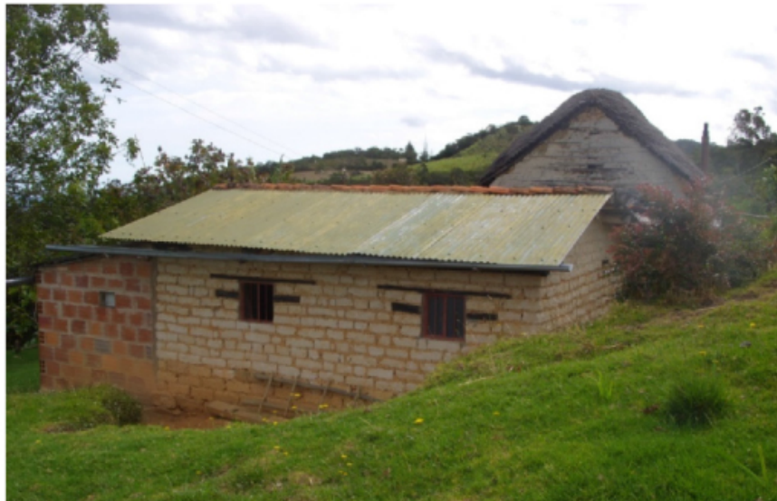
Figure 52: Adobe masonry Source : MATERIALITY OF RURAL VERNACULAR HOUSING IN THE ANDEAN HIGHLANDS OF COLOMBIA: ENVIRONMENT AND BUILDING SYSTEMS www.witpress.com , ISSN 1746-4498 (on-line)
