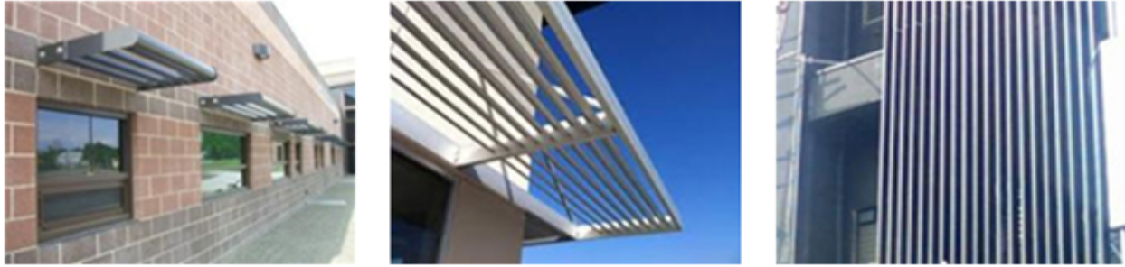
Figure 50: Aluminum architectural sun shade, horizontal sun control device, vertical fins
