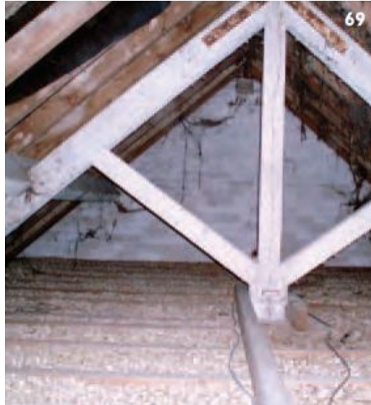
Figure 32: A typical ‘cold roof’ insulated with vermiculite between the ceiling joists © Oxley Conservation (bui)
