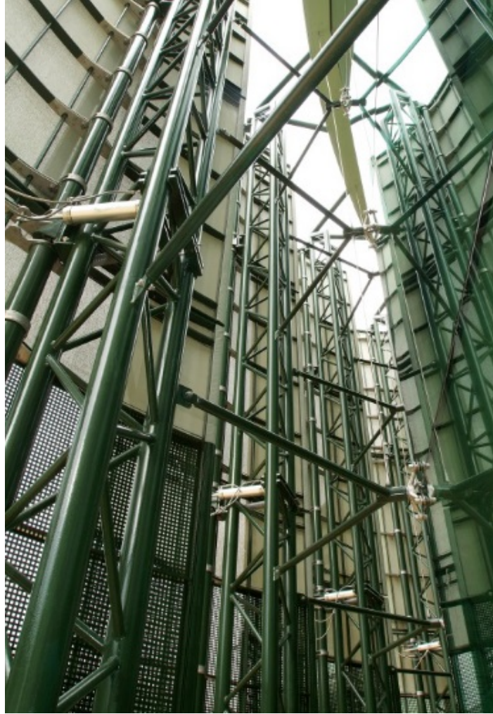
Figure 60: The thermo-hydraulic drivers animating the fins
