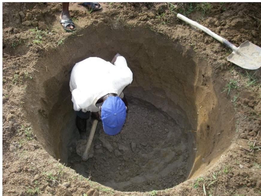
Figure XII Spading Shallow Wells
