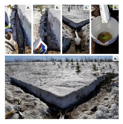
Figure 2: Figure 2. Runoff collector construction phases. a) Two 10-15 cm trenches were dug into the frozen ground, b) hydraulic cement was used to seal the garden edging into the trenches, c) trenches tapered at the bottom of the slope to form a "V" where an eavestrough was used to funnel water towards the bucket with a v-notch, d) a pressure transducer was used to continuously measure water height and discharge, e) completed runoff collector where each arm of the "V" was ~4m.
