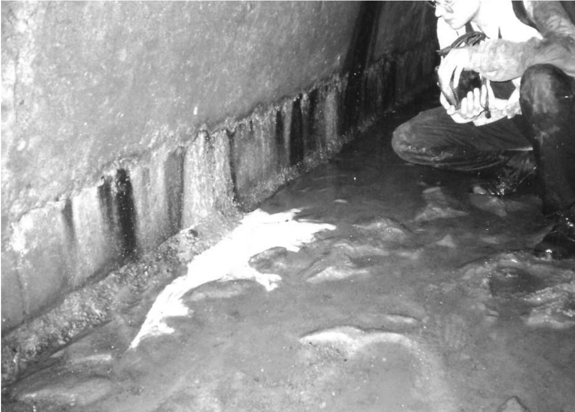
Fig. 3b. Spring issuing from fissure in the Washington Avenue tunnel. Seepage entrains whitish St. Peter sand grains from outside the tunnel lining. Photo by author.
