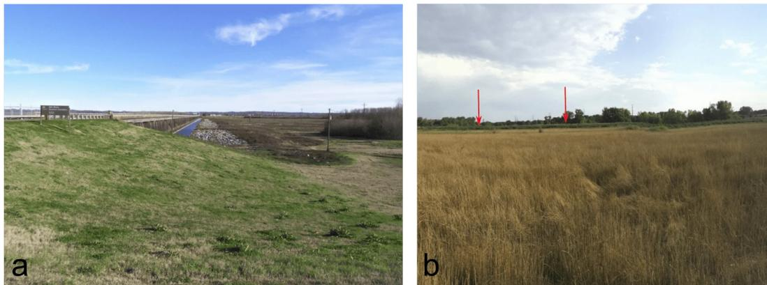
*Figure 14. Two artificial levees in the NLD. (a) Over 7 m high, a massive levee west of the overbank structure at the Old River Complex, Louisiana, USA. (b) Almost invisible, Fort Collins North- Cache La Poudre River, ~1 m high, Colorado, USA, indicated by two arrows.*
