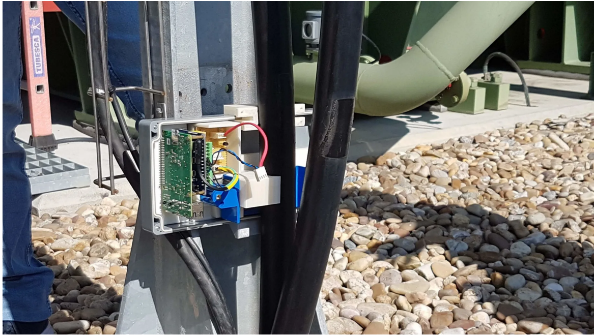
Figure 3: Photo of the sensor installed at SPI substation, clamped around the transformer TFR6 neutral grounding cable.
