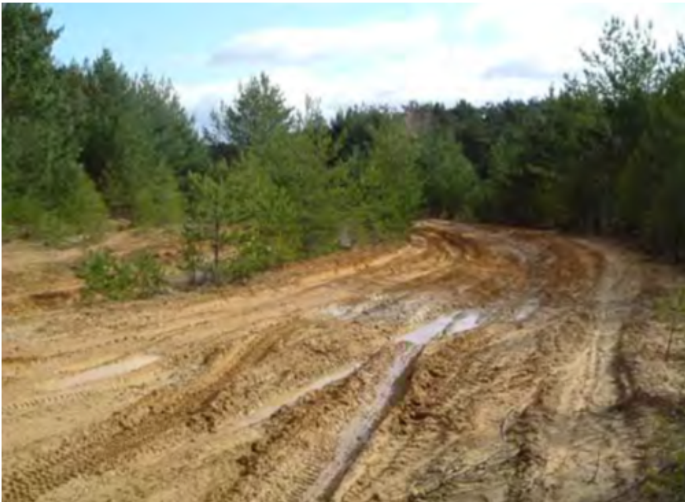
Figure 10. Hydraulic action by vehicles within depressions and standing water
