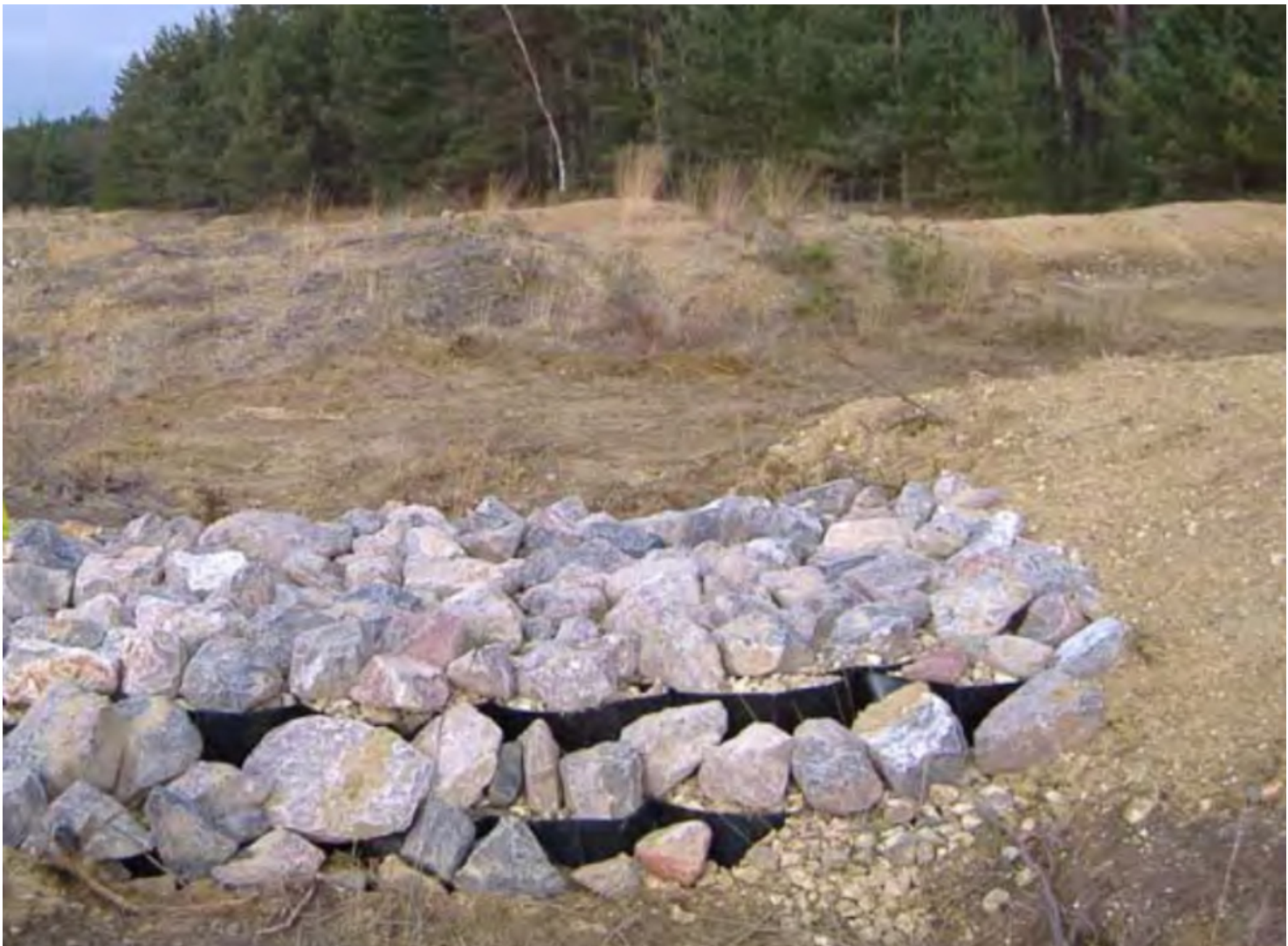
Figure 24. Use of cellular geotextiles and coarse sediment to trap fine sediment
