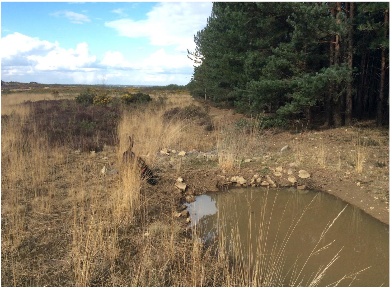
Figure 26. Stone filled gabion deflectors to promote deposition and divert flow paths
