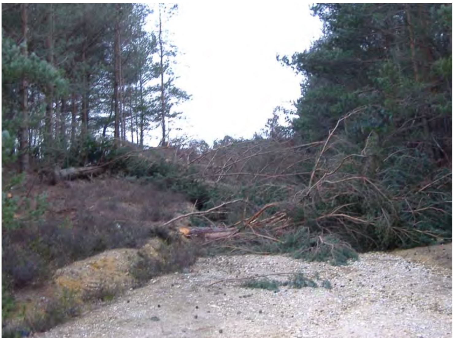
Figure 21. Buried felled tree used to form flow deflector on wide track (flow diverts from left to right)
