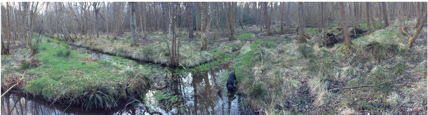
Figure 29. Diversion channels and embayments for sediment deposition
