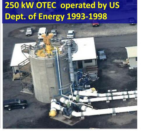
Three land-based demonstration OTEC plants are operating now in Hawaii, near Okinawa, and in South Korea. These plants generate power onto the grid day and night and are sited near steep seafloors with 3-km access to deep cold water.
